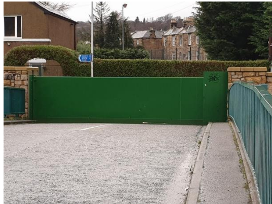
Floodgate on Saughtonhall Bridge, Dec 2020
